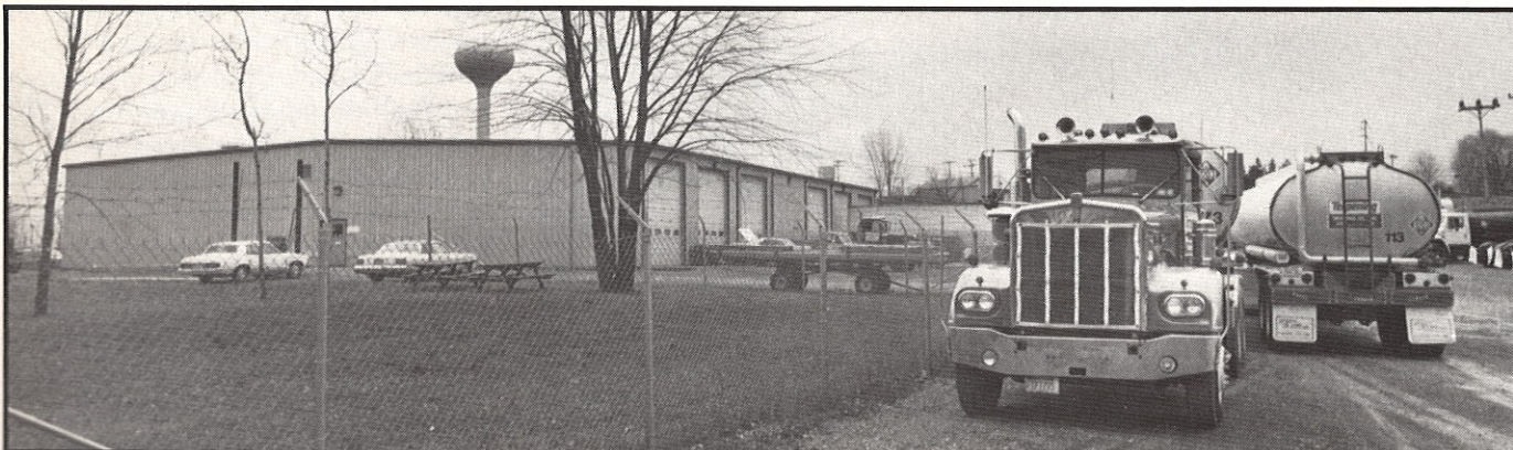
Terpening Trucking and Utility/Tri Tank are located on a 24-acre site off I-90 and I-690 in Syracuse NY. The companies share the 140-ft by 110-ft building constructed in 1984. About 70% of Terpening Trucking's revenues come from local transportation of gasoline and aviation fuel.
